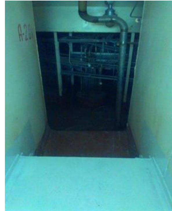
Concrete barrier in the melt spreading area to avoid containment bypass (WWER-1000/V-302 peculiarities)
